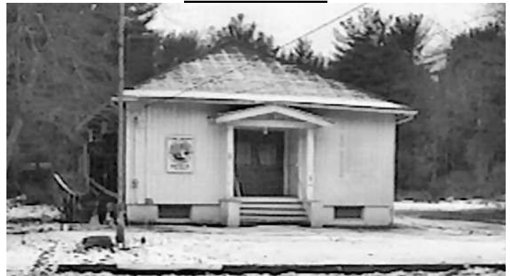
The former Chapter 36 Building , located in Middleboro.
